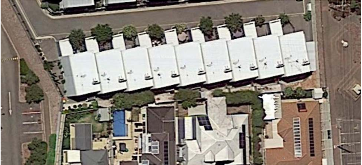
Figure 1. Roof-mounted air conditioning units approved at 3 Barwell Avenue, Seacliff
