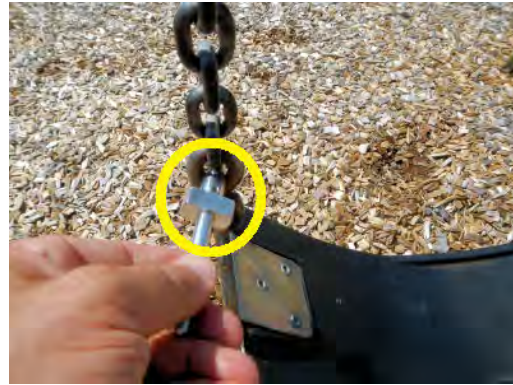
Photo taken: 28/11/2016 S-hook openings=10mm on both swings.
