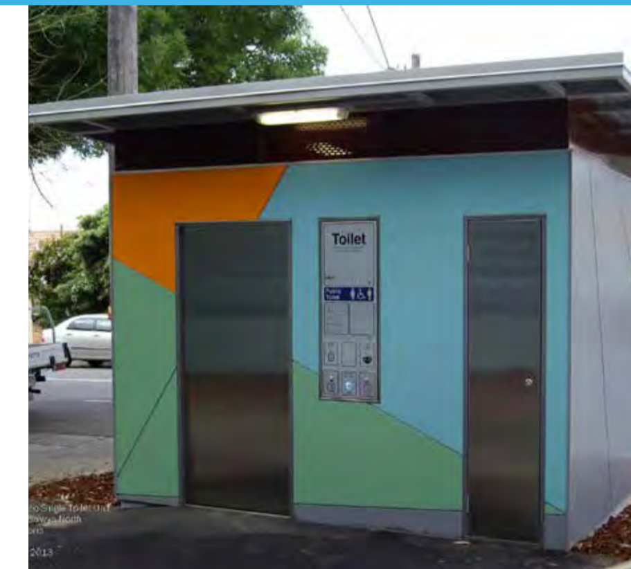
EXELOO TOILET - AUTOMATED ACCESSIBLE TOILET WITH 1 x ADULT CHANGE TABLE
