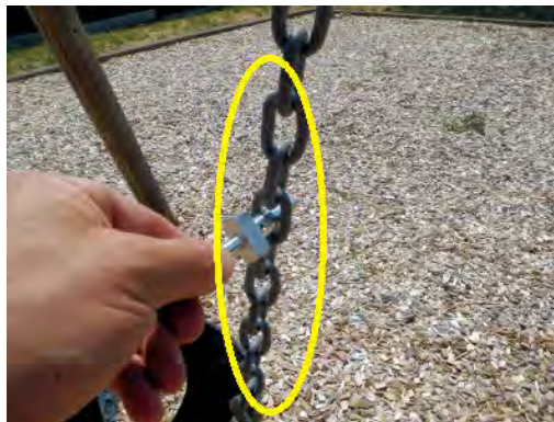
Photo taken: 28/11/2016 Toddler swing chain and connection openings=10mm.
