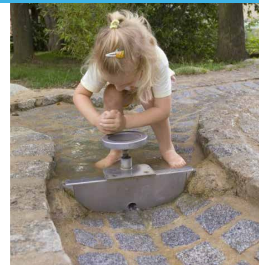
WATER PLAY CRANK GATE - LOCATED WITHIN SWALE TO ENABLE WATER COURSE MANIPULATION
