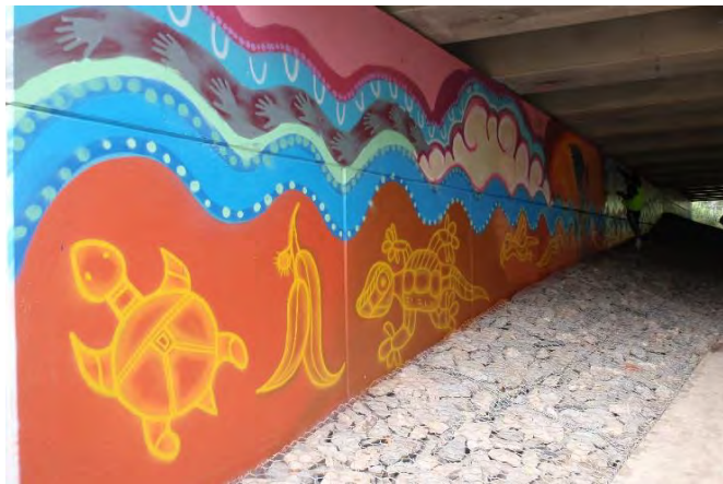
Warriparinga Walk Mural Souther Expressway bridge, Warriparinga
