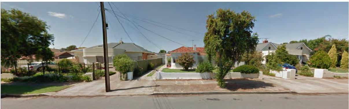
Figure 41. 3 original dwellings used as semi-detached dwellings in Elder Terrace
