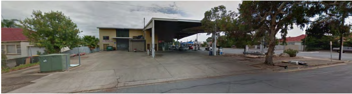
Figure 13. View of the land from Cungenya Ave (2-storey scale on boundary)
