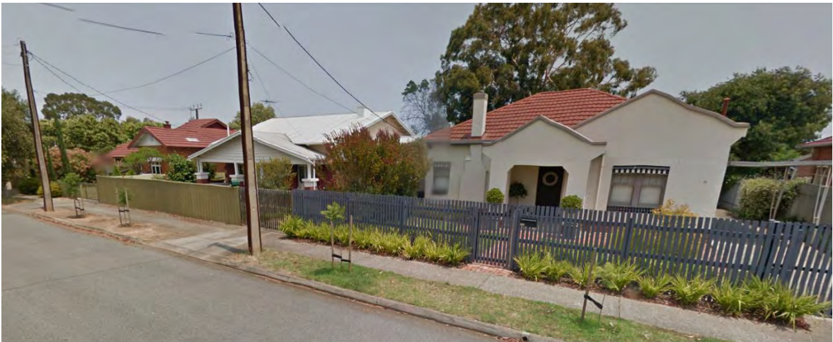
Figure 22. Housing stock in Arthur Street
