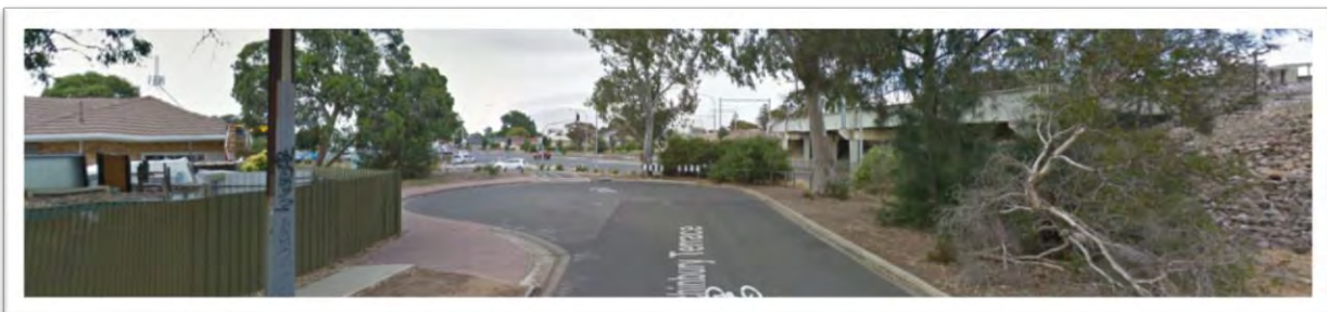
Minchinbury Tce – eastern end – Rail corridor embankment and bridge over Marion Road are dominant features
