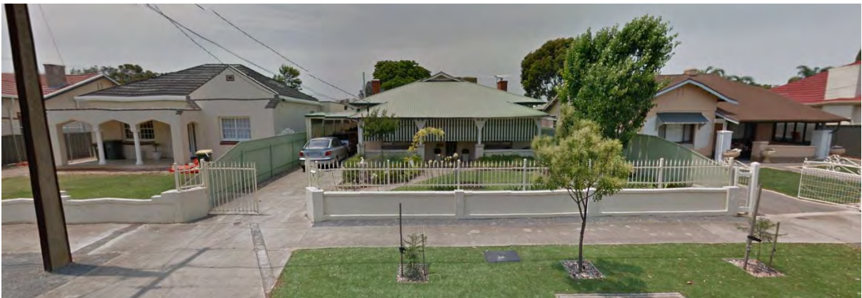
Figure 23. Housing stock in Arthur Street
