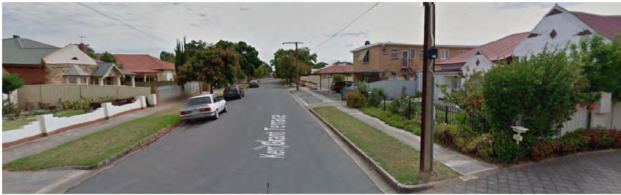
Figure 34. Kerr Grant Tce (northern end) – 1960s 2 storey units amongst predominantly original housing stock
