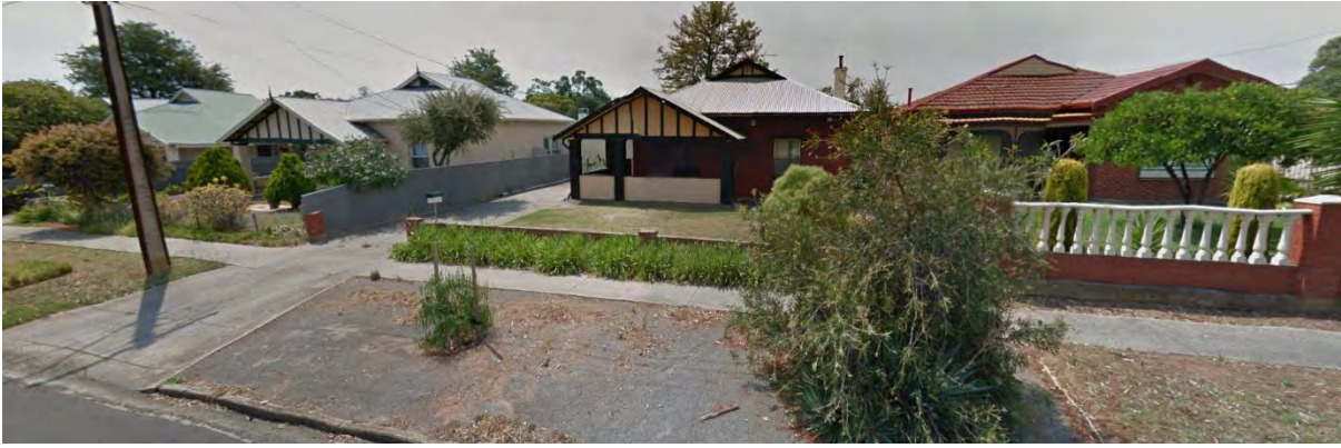
Figure 16. Bungalows along Wright Street
