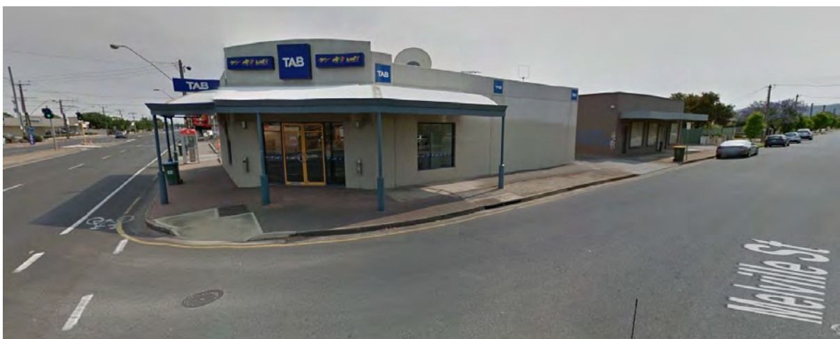
Figure 2. The site viewed from Melville Street
