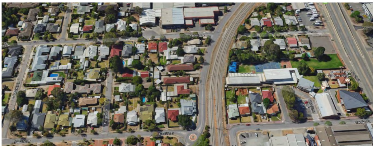
Figure 15. Consistent street tree planting is not evident
