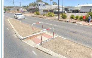
Mid-Block Pedestrian / Cycling Refuges and Kerb Ramps
