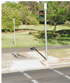
Bicycle/Pedestrian Activated Crossings (PAC/BPAC)
