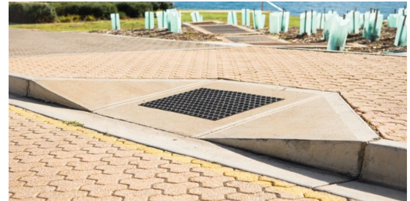
Figure 6: Kerb Ramp in Hallett Cove
