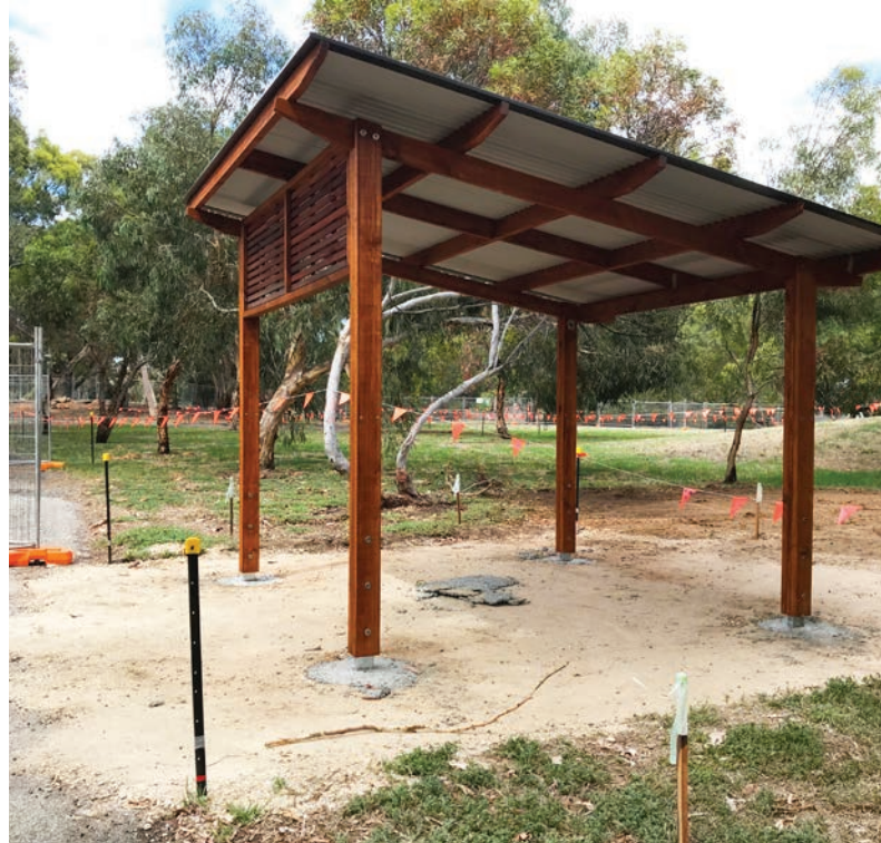
▲ Installation of additional small shelter near Japanese garden
