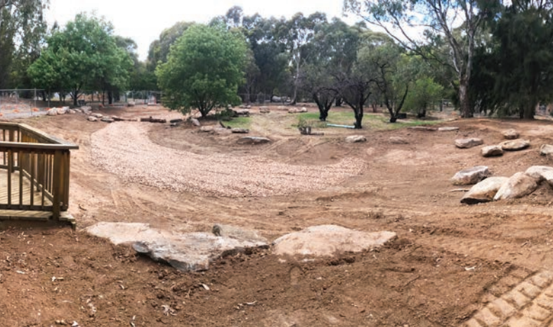
Dryland creek under construction ▲
