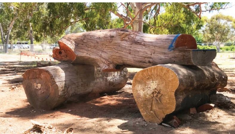
Construction of nature play timber climb using old logs from site ▲
