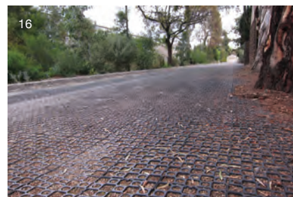
Pervious surface on section of the road adjacent significant native trees Charles Lane, Unley
