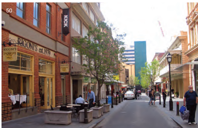
Leigh Street, City, Adelaide (V-C) One-way traffic street has a shared single surface in the middle section, vehicular path separated by spoon drains and street furniture (lamp columns, planters, bins and bollards and popular destinations including cafes, restaurants and offices)
