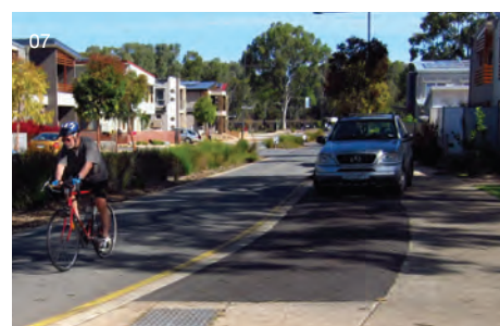
Horizontal deflection (bending road) and visual carriageway narrowing through landscaping Lochiel Parkway, Campbelltown, Adelaide
