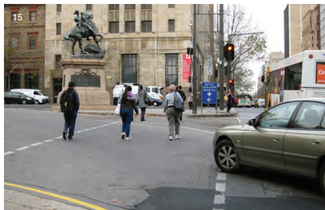
15 Car priority at slip lines with cars able to turn left into pedestrian path at any time, Intersection North Terrace and King William Street, City, Adelaide
