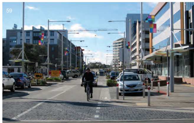
Rumble strips at intersections raise awareness of vehicular speeds Childers St, Canberra
