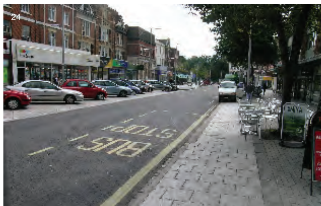
London Road, Southampton (IV-C) Neighbourhood collector road in a district activity centre with asphalt carriageway and paved pedestrian areas (also accommodating angled car parking)
