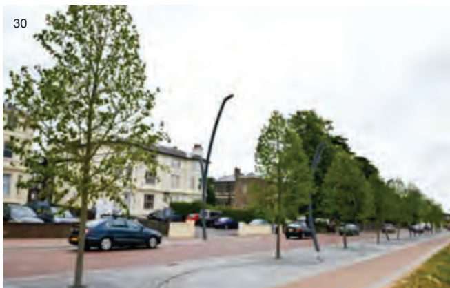
30 Elwick Road, Ashford (UK) (II-D) City centre of Ashford, including ring road carrying over 10,000 vpd, redesigned as a shared level surface environment with distinct pavement patterns and stormwater treatment
