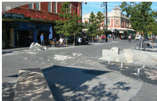
Hargreaves Mall, Bendigo, NSW (IV-A) Shared level surface city centre mall carrying c.3,200 vpd includes rumble strips, water features and unlined two-way carriageway spaces
