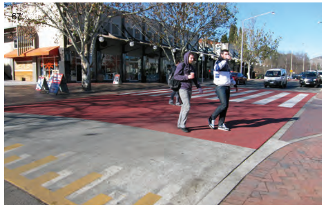
67 Raised carriageway profile at crossing points Flinders St, Manuka, Canberra
