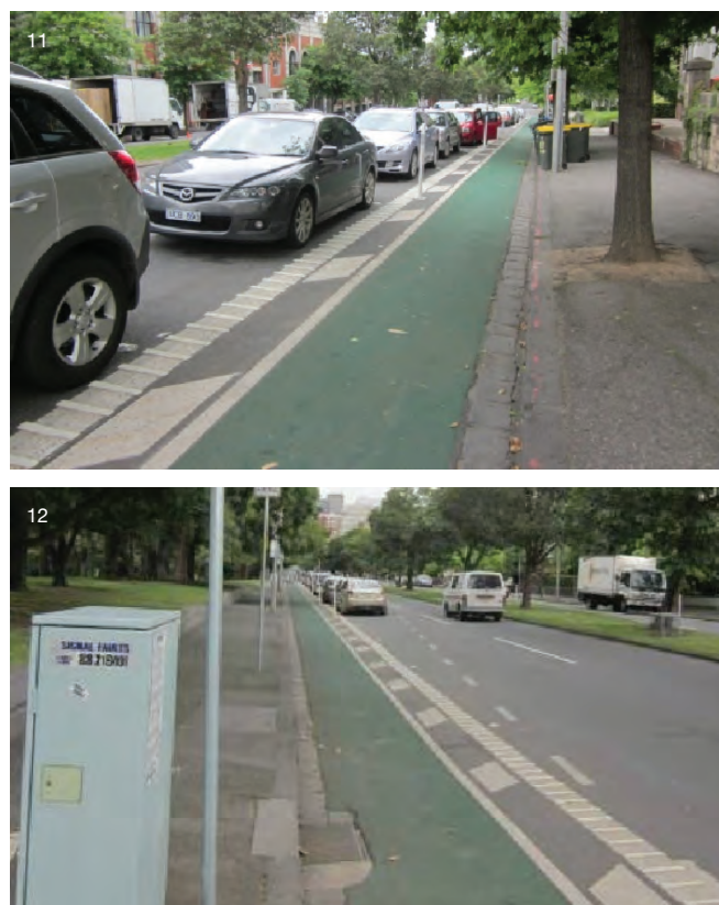
Figure C10. Cyclists incorporated between pedestrian and car parking spaces Albert Street, East Melbourne
