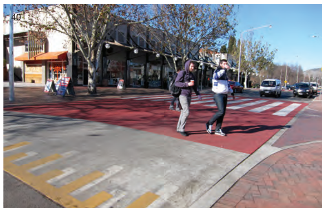
Bouganville Street, Manuka, Canberra, ACT (IV-B) Busy mixed-use centre in Canberra with at-grade crossing points and side road entry treatments
