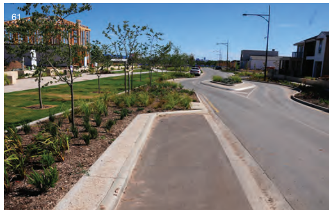
61 Horizontal deflection (traffic island bending the car path) and visual carriageway narrowing through landscaping Lightsview, Adelaide
