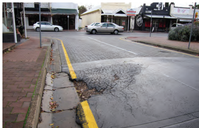
Poor road surface within a metre of the kerb, Thomas Street, Unley, Adelaide
