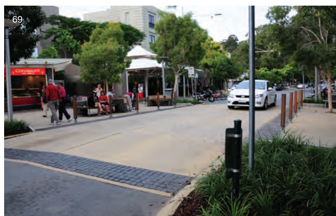
69 Reduced carriageway width at pedestrian crossings Hastings Street, Noosa
